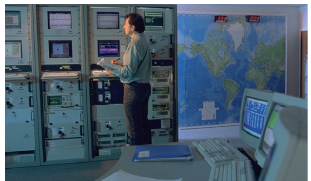
Using state-of-the-art independent control centres
